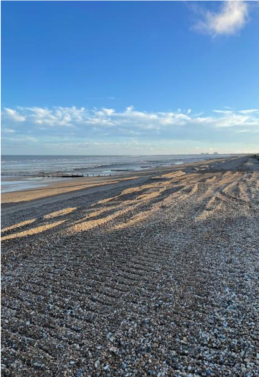
Winter coastal defence work at Littlestone Beach
