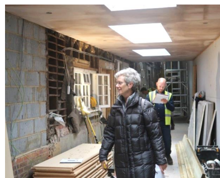
Photo: Helen reviews progress in the foyer.
